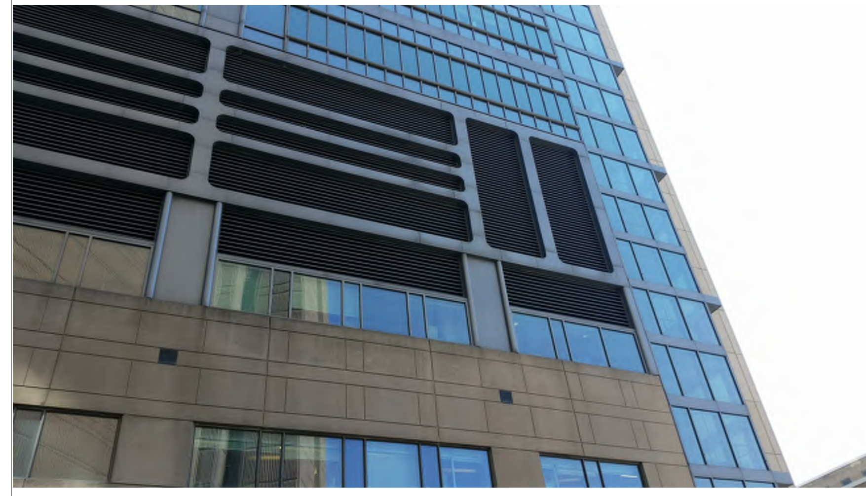
6 PMC EXTERIOR PHOTOGRAPH A80-00-02 N.T.S.
